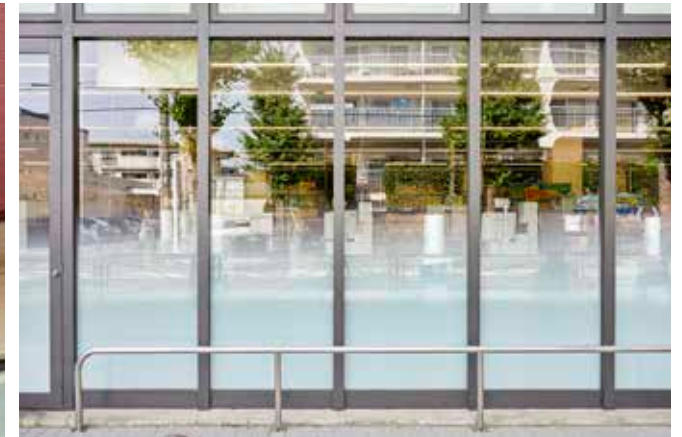
From the outside of the building
